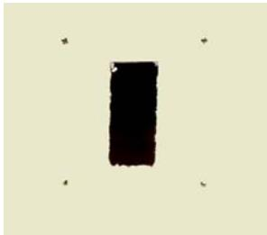
**Fig.7:** The four (4) outside mounting holes have been marked and the rectangular center opening has been traced and removed from the wall. The four (4) drywall anchors have been inserted into the wall.
